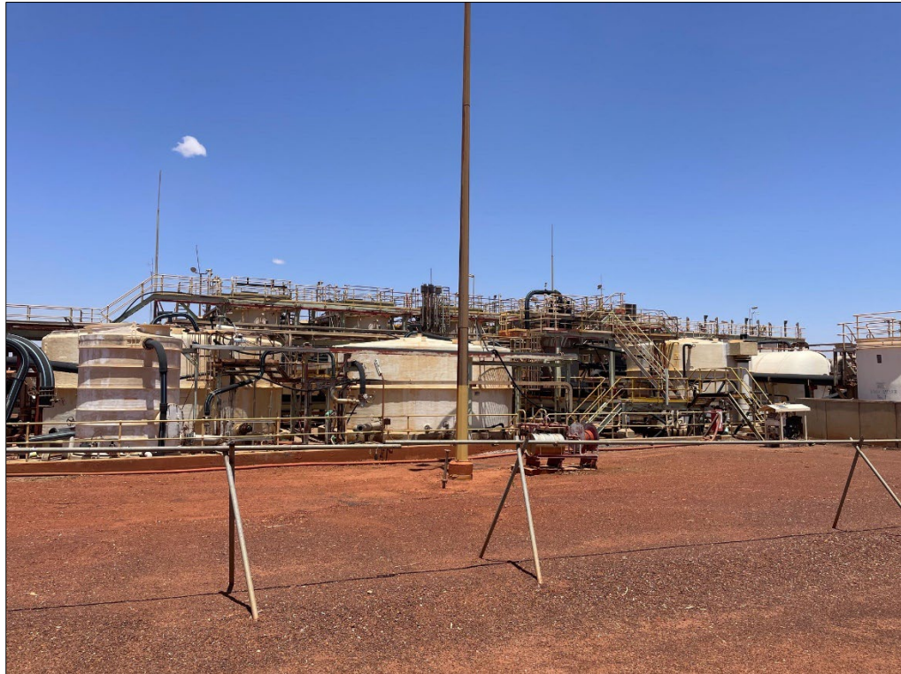
Figure 9-3: Solvent extraction plant
